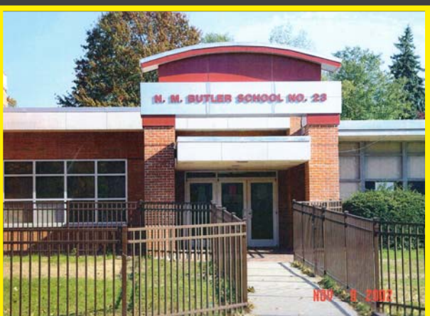
Butler School Repair
