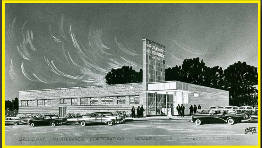
Broadway Maintenance Corporation (1969)
